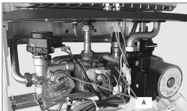
**Attention. When reassembling the exchanger be sure to put the off center location/securing pin indicated towards the left side of the boiler.**
