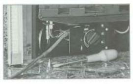
If the setting pressure is too low, but the meter pressure is acceptable, then a problem in the supply pipework is to be suspected. This will be dirt and debris, kinked or inadequate size pipes, restriction in a fitting or solder flashing across a joint.
