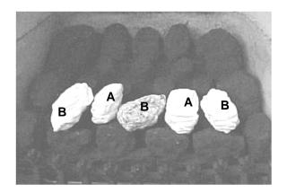
Lay second row of loose coal 3 off "A" and 2 off "B" coals as shown so that they rest on the high projections of the BASE MATRIX behind the previous row.
