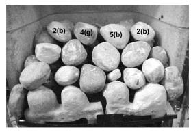
Lay the three remaining loose pebbles as shown.
