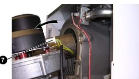
Remove the inspection hatch, fan, burner and gas block unit.
