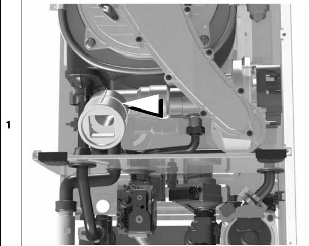
Isolate the gas supply. Disconnect the gas pipe.
