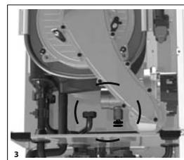
5. Disconnect the gas supply from the venturi assembly (fig 3)
