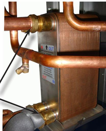
*Remove screws from either side of plate heat exchanger*
